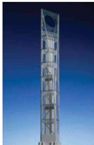
The Outriggers are effectively act as stiff headers inducing a tension-compression couple in the outer columns.
